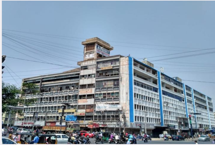
Structural stability test for Chandralok complex
