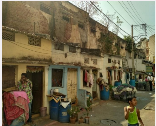
Structural Stability test for row of houses Kachiguda, market back side.
