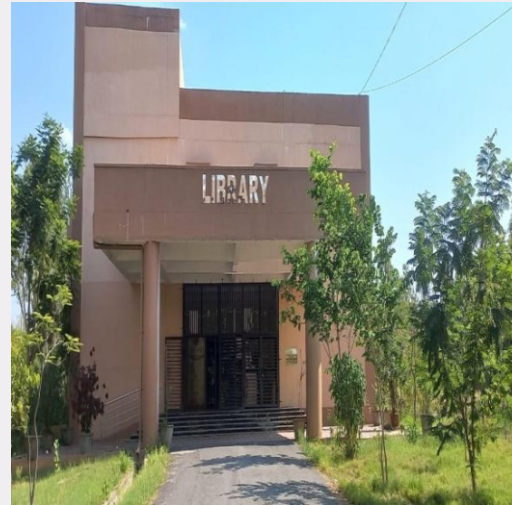
LIBRARY BUILDING AT JNTUH, MANTHANI
