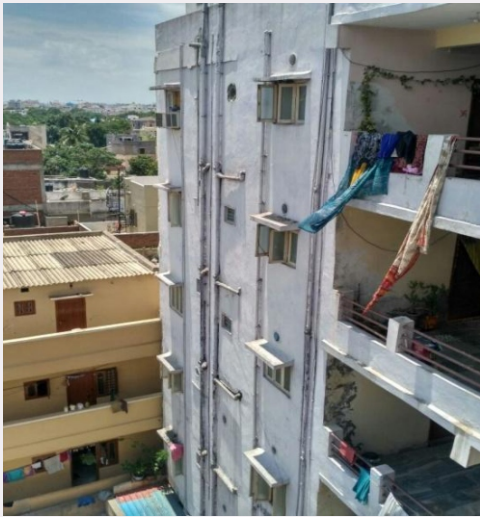
Structural stability test conducted at Sunder Nagar, at Sajjan Lal Street, Monda
