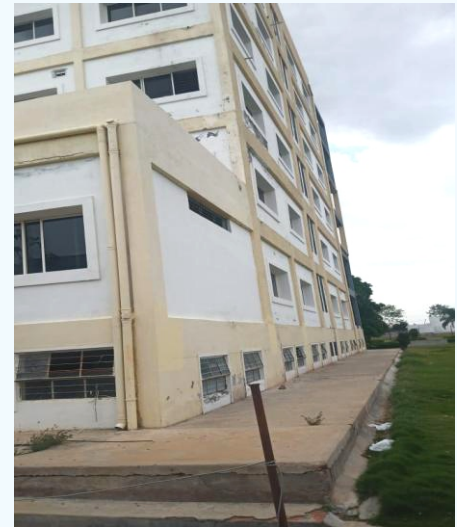
Structural Stability test for Sphoorthy Engineering College, Hyderabad
