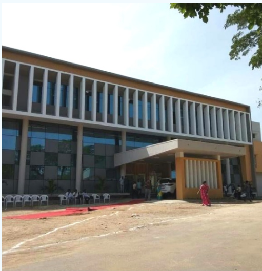
Proof checking of Indoor stadium, JNTUH
