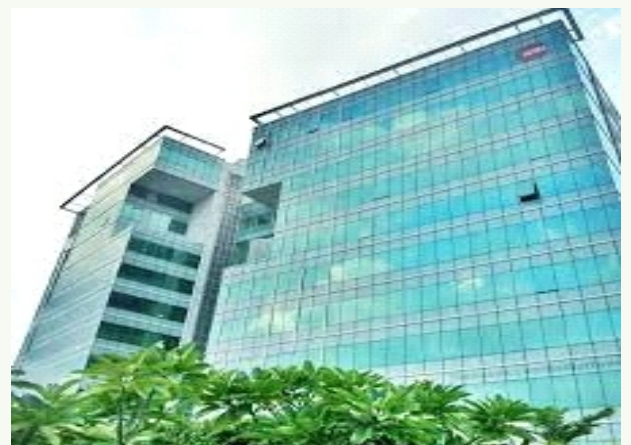
Structural Stability testing of existing building at Sri Ram Nagar Colony Patancheru
